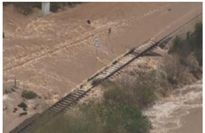
Flooding at Cowley Bridge rail line, November 2012 (Source: ITV News).
